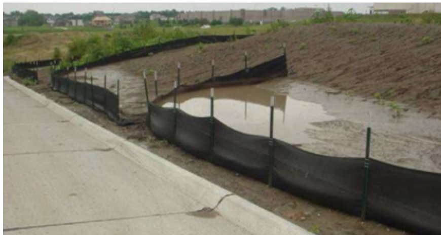
Figure 12: Typical Example of a Silt Trap fence
