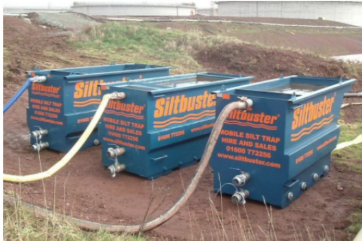
Figure 11: Typical Example of Settlement Tanks
