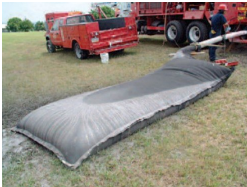
Figure 10: Typical Example of Silt Bag
