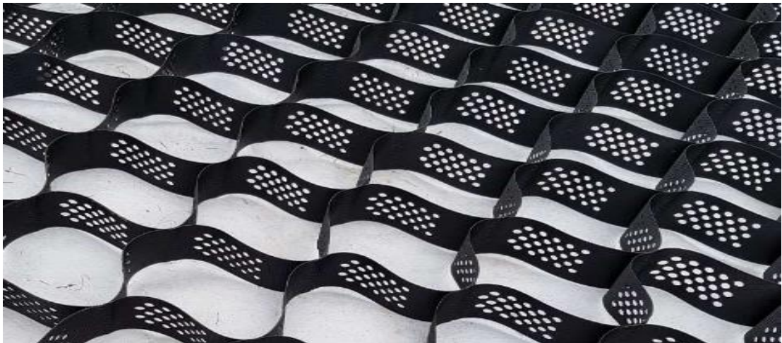
FIG. 1 – Expanded geo-cell sheet prior to been filled with angular stone
